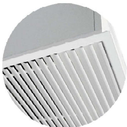
Detail of exposed inlet grille
